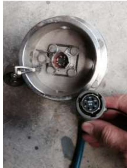
Figure 8: Pressure Transducer Connection
